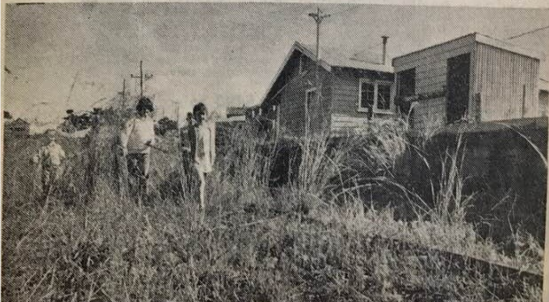
1971. Paper clipping: Belmont Derelict Railway Station.
