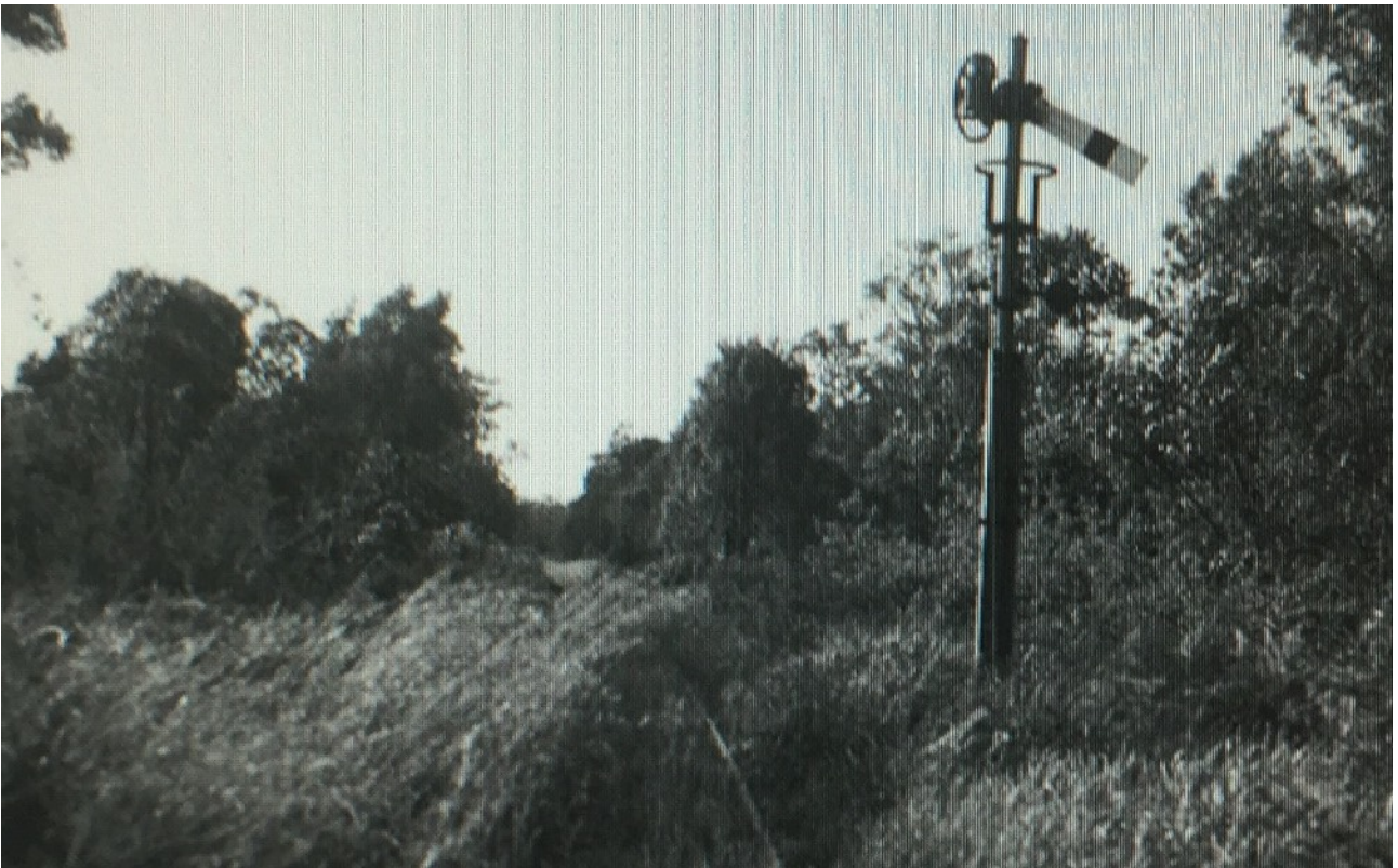
1971. Disused Belmont Railway line.
