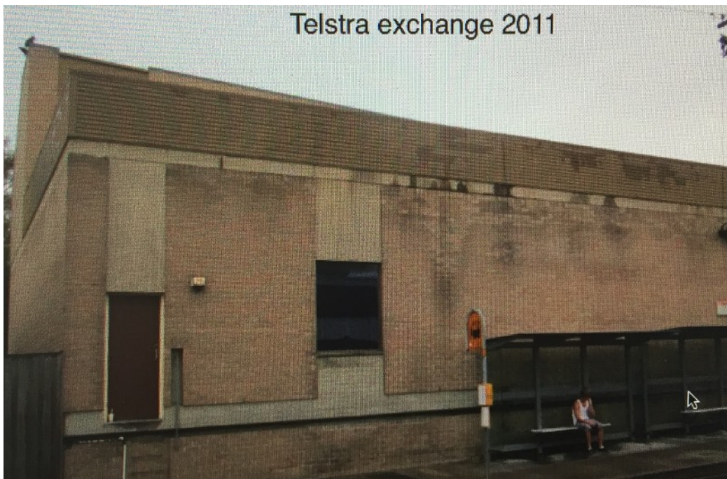
Telstra Exchange Pacific Highway Belmont.
