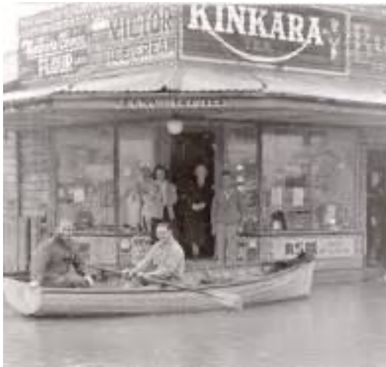
1949. 18th June. Marks Point flood - shop and Post Office.
