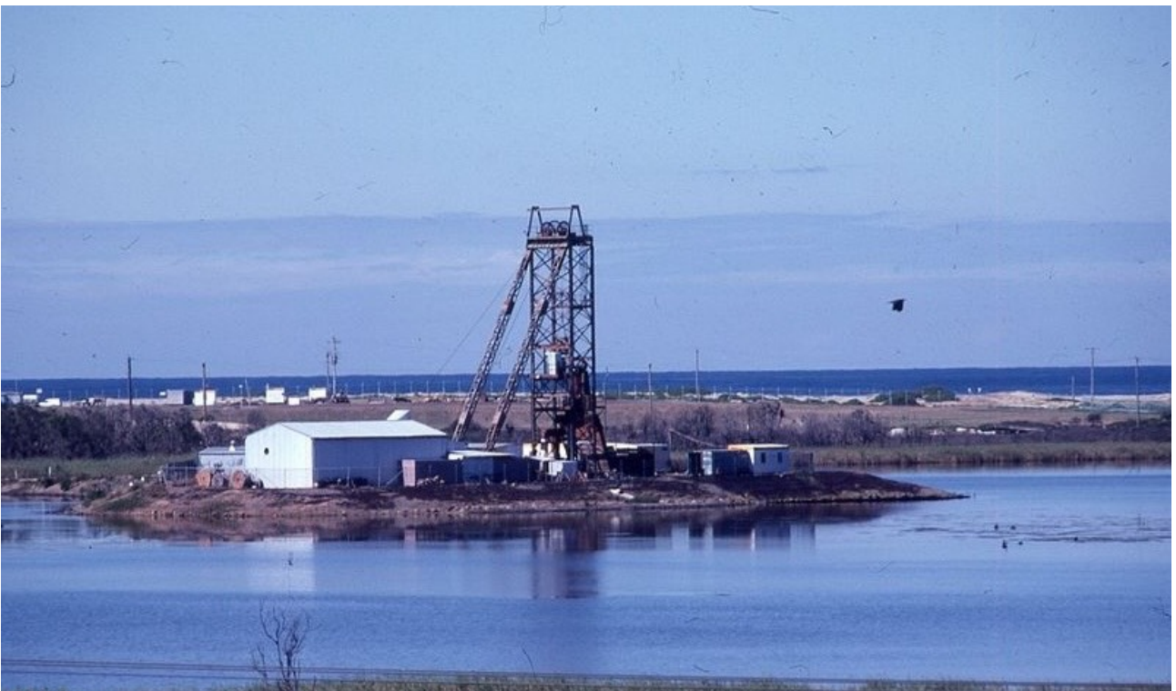
1982. Sinking head frame for John Darling Colliery N04 shaft Belmont Lagoon May 1982.
