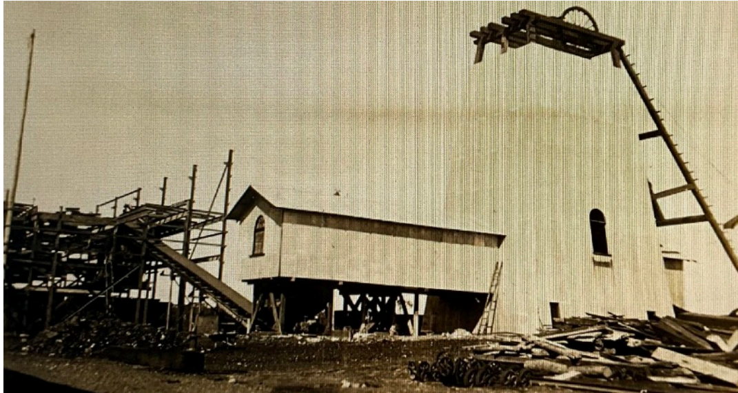
1928. John Darling Colliery, Belmont, Lake Macquarie, NSW. No.2 shaft (upcast) with temporary Headframe.
