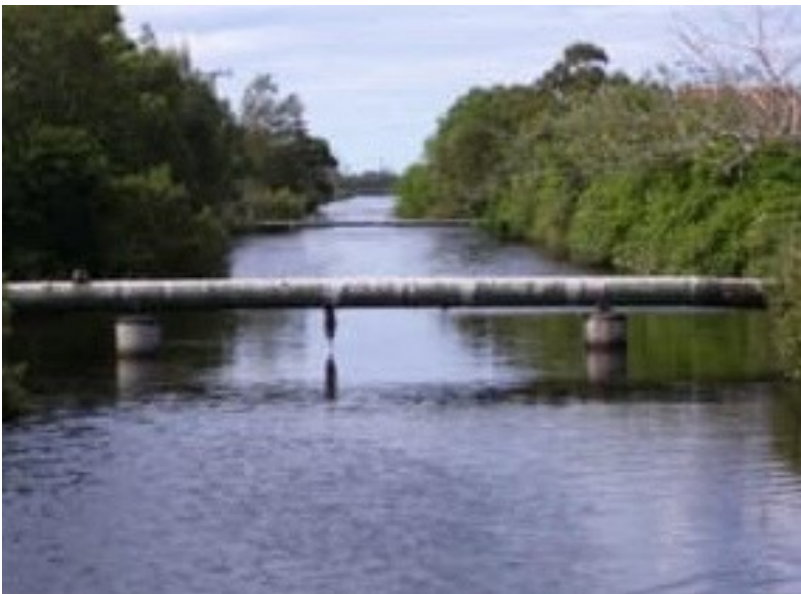
Cold Tea Creek (Anti Tank Ditch)
