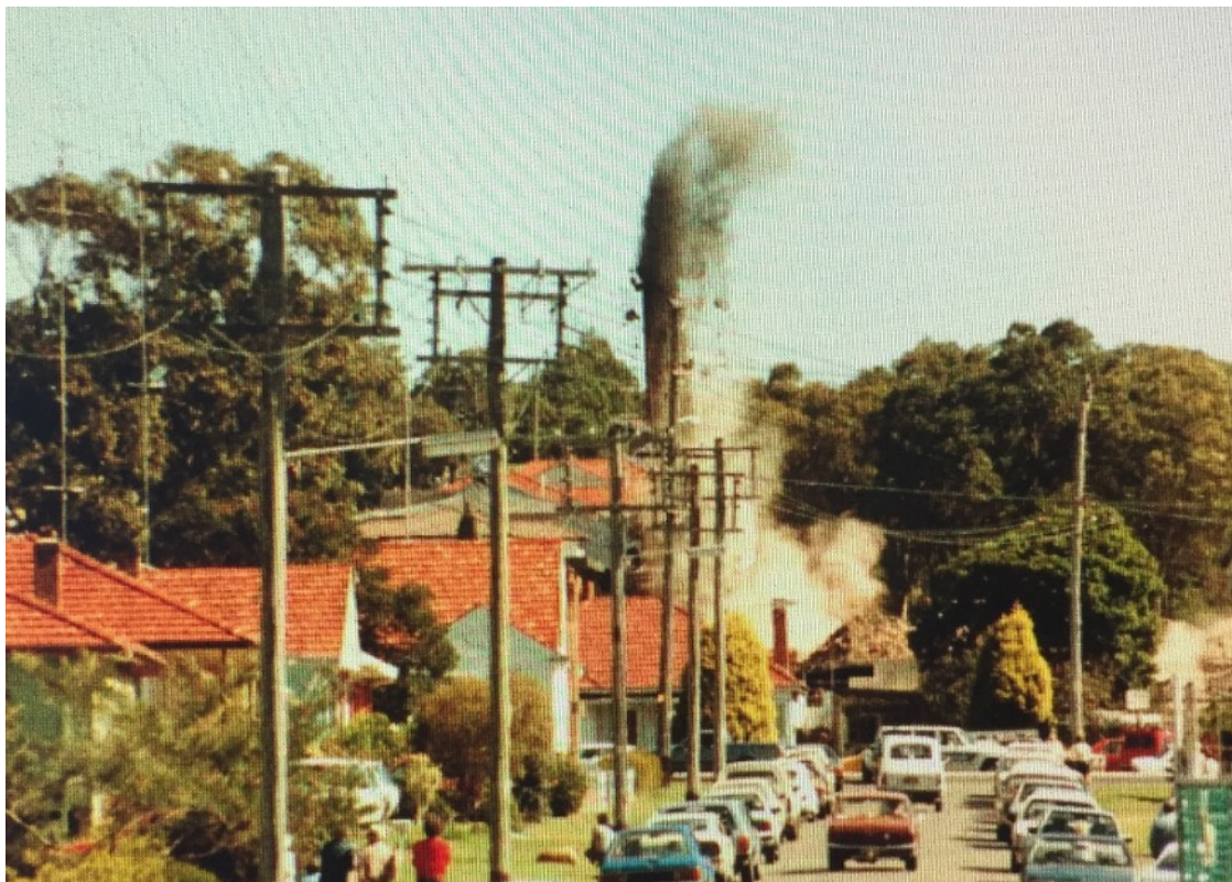
1970's. Demolition of Belmont Pipe Works.
